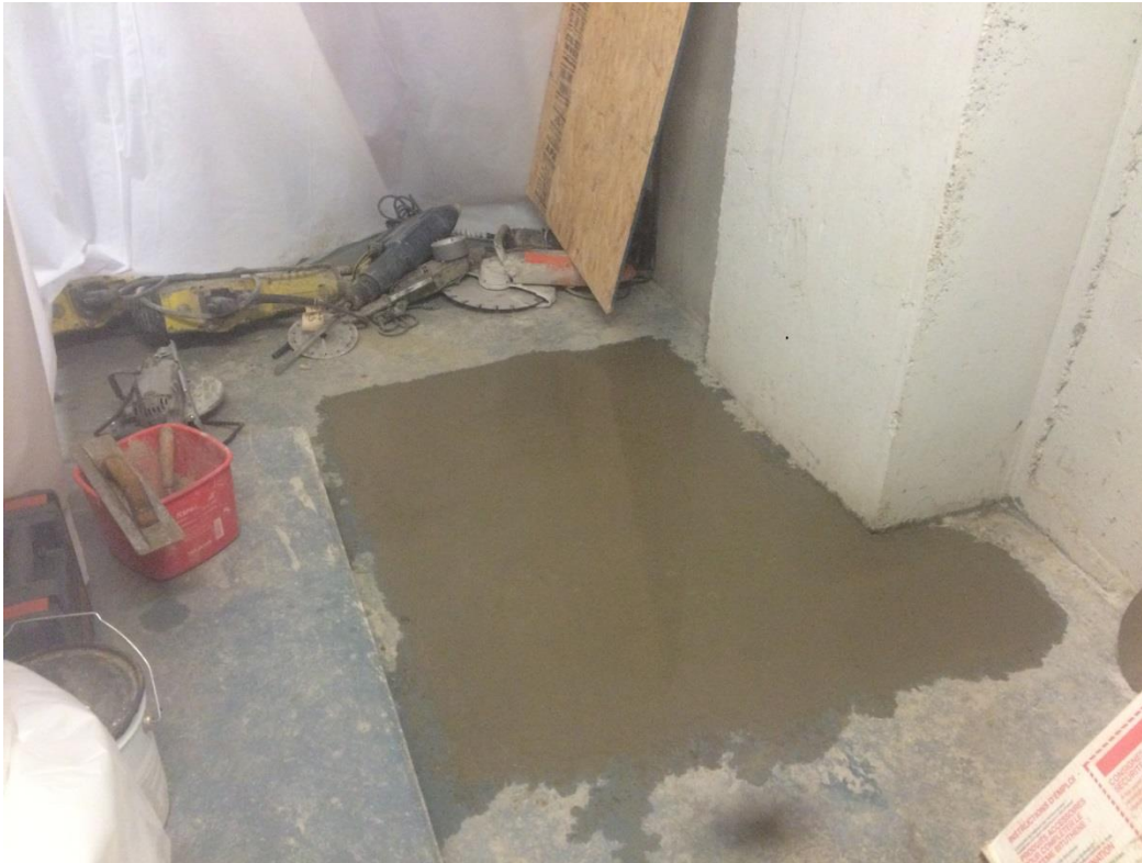
Photo No. 18 – Test Pit TP-5: Backfilled, compacted and grouted (facing south)
