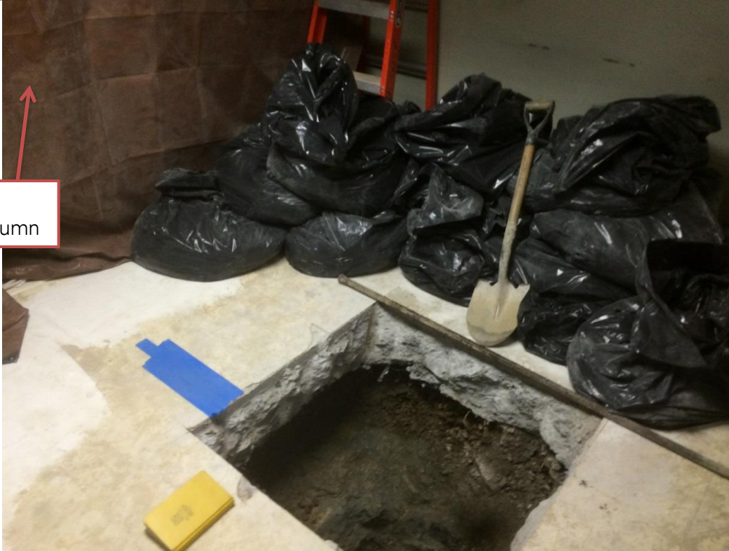
Photo No. 1 – Test Pit TP-1: General view (facing south-west)
