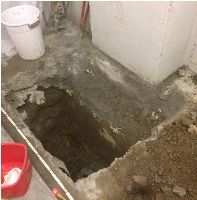
Photo No. 16 – Test Pit TP-5: Backfilled, compacted and grouted (facing south)
