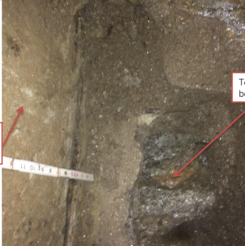
Photo No. 17 – Test Pit TP-5: Backfilled, compacted and grouted (facing south)
