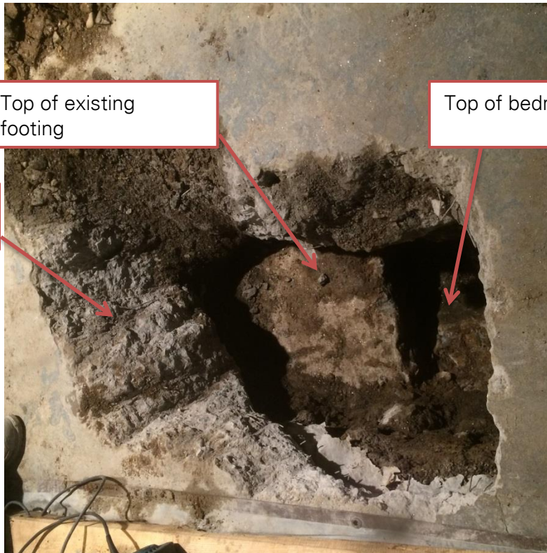
Photo No. 10 – Test Pit TP-4: View of top of existing footing
