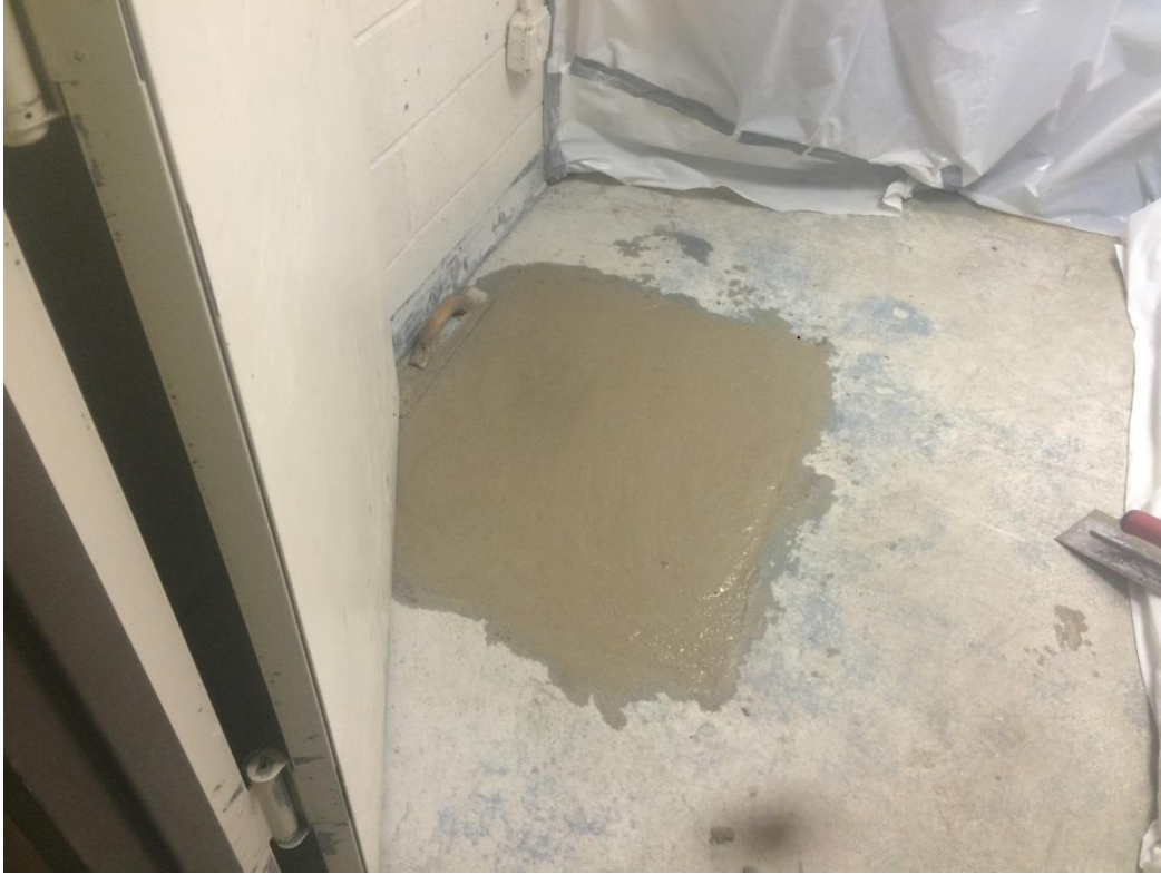
Photo No. 14 – Test Pit TP-5: Backfilled, compacted and grouted (facing south)
