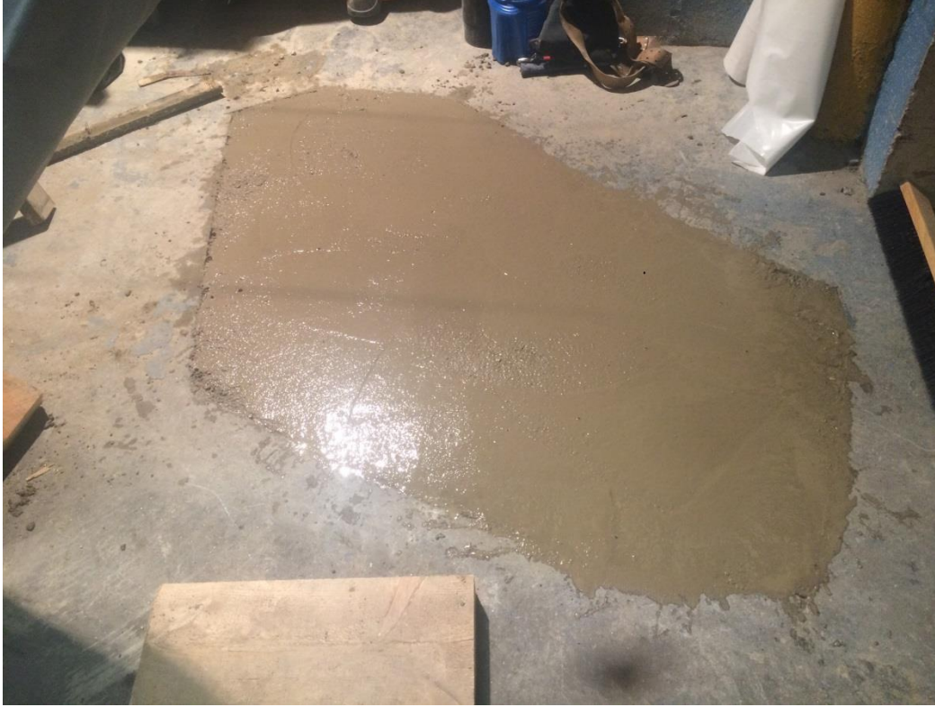
Photo No. 11 – Test Pit TP-3: Backfilled, compacted and grouted (facing south)
