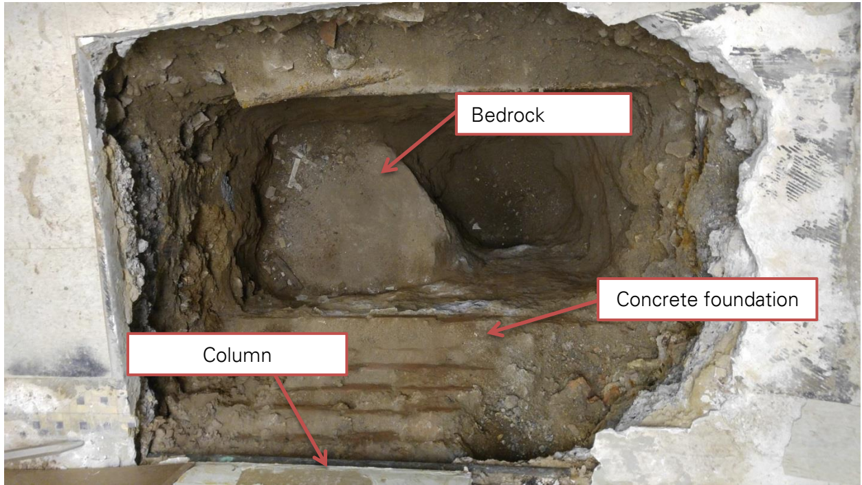
Photo No. 5 – Test Pit TP-2: View of foundation (facing north)
